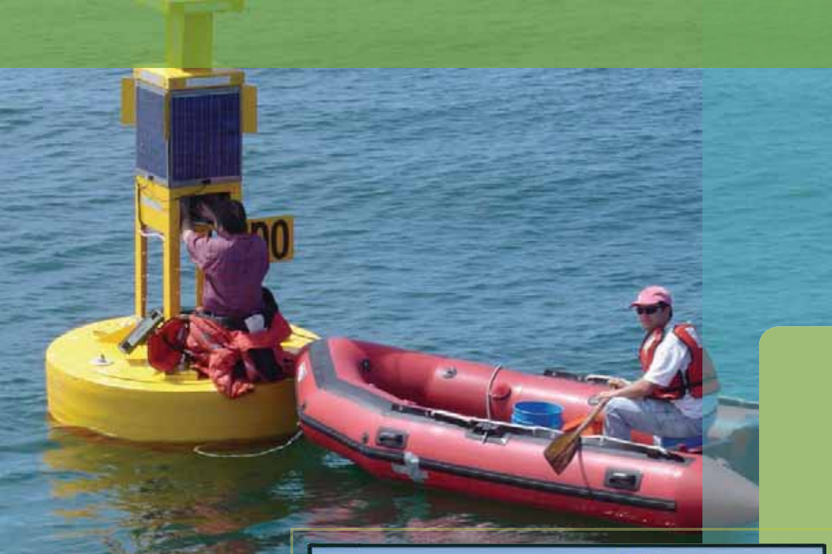
Above: OHSU field staff members Michael Wilkin and Jon Graves rewire an ocean observing buoy on a calm day in the Pacific Ocean west of Seaside, Oregon. Photo: Courtesy of CMOP
