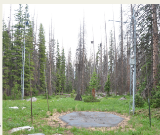
Brooklyn Lake SNOTEL site, WY. From left to right: antenna with temperature sensor, solar panels; snow pillow and ground truth markers; precipitation gauge (pressure transducer); snow depth sensor (radar).
